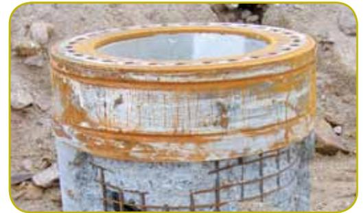
Traditional pile foundations can suffer severe damage in extreme ground conditions
