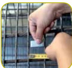
③ Short glued fibres are clearly the fibres of choice to reach homogenous reinforcement without fibre blocking between the rebars.
